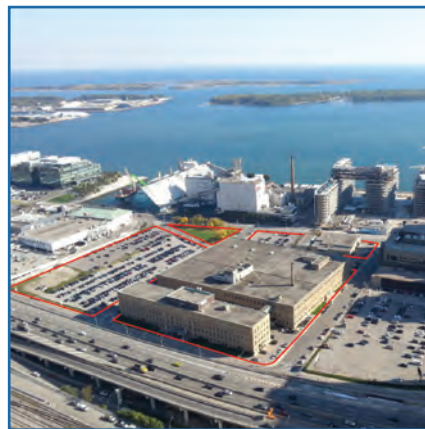
LCBO - Head office Redevelopment
